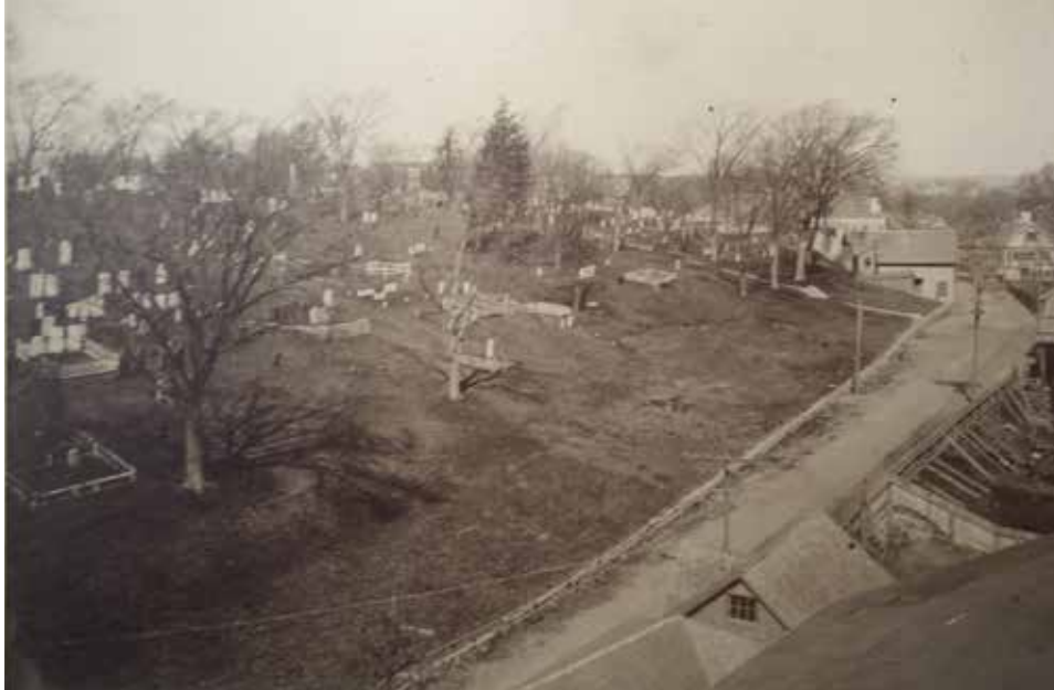
Figure 7. Photograph taken after the demolition of the stable buildings and school on School Street, looking north, before the area had been fully filled and graded.
