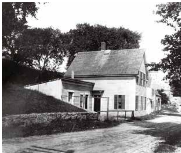
Figure 10. Photograph of houses along School Street, showing how they were cut into the hillside (Baker and Keith 2013: 8).
